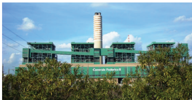
Enel Federico-II thermoelectric power plant
