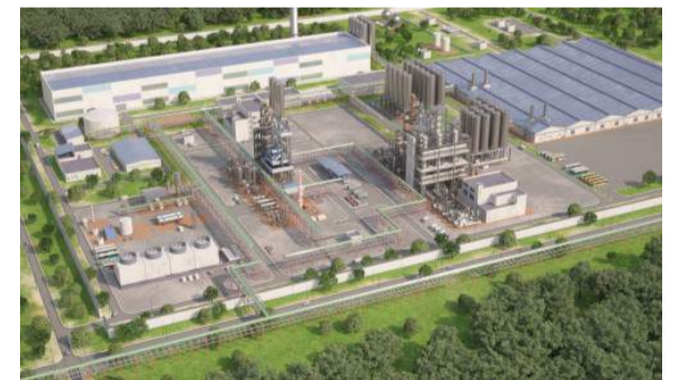
Sumgayit SOCAR polymer plant project
