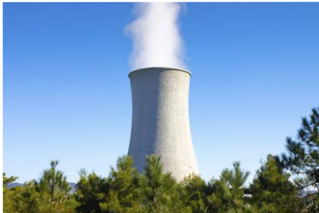
Sasso Pisano geothermal power plant- cooling tower
