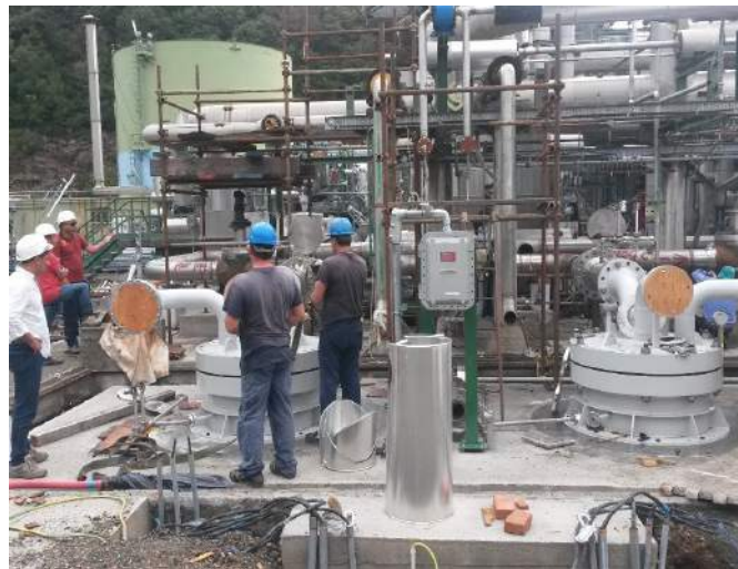
On-site pump installation by TMP
