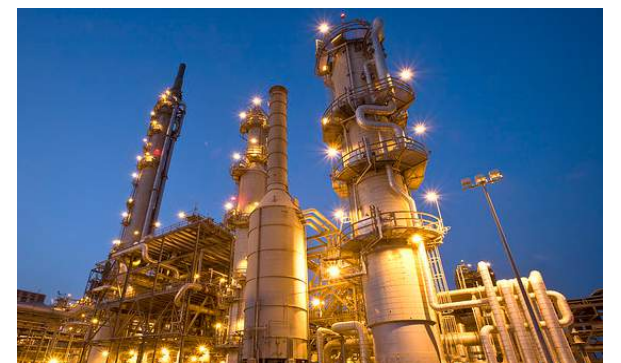
Petrochemical plant – ammonia production plant
