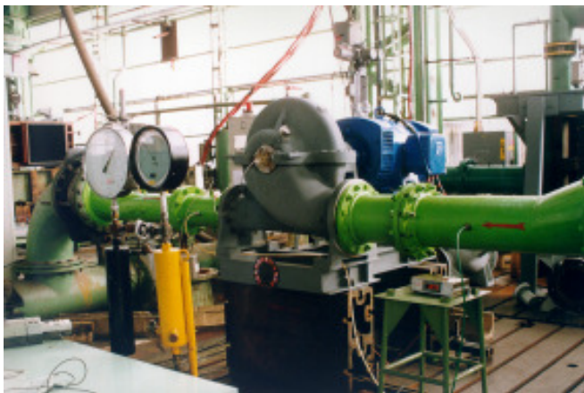
HSS pump during testing at TMP test Center
