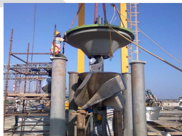
Impeller installation
