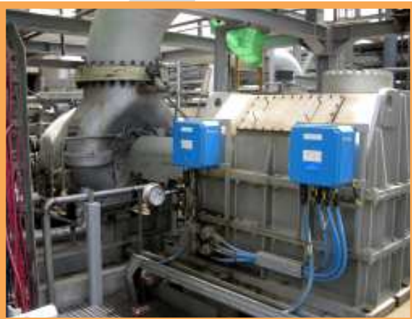
Turbine and reduction gear with angular take-off shaft
