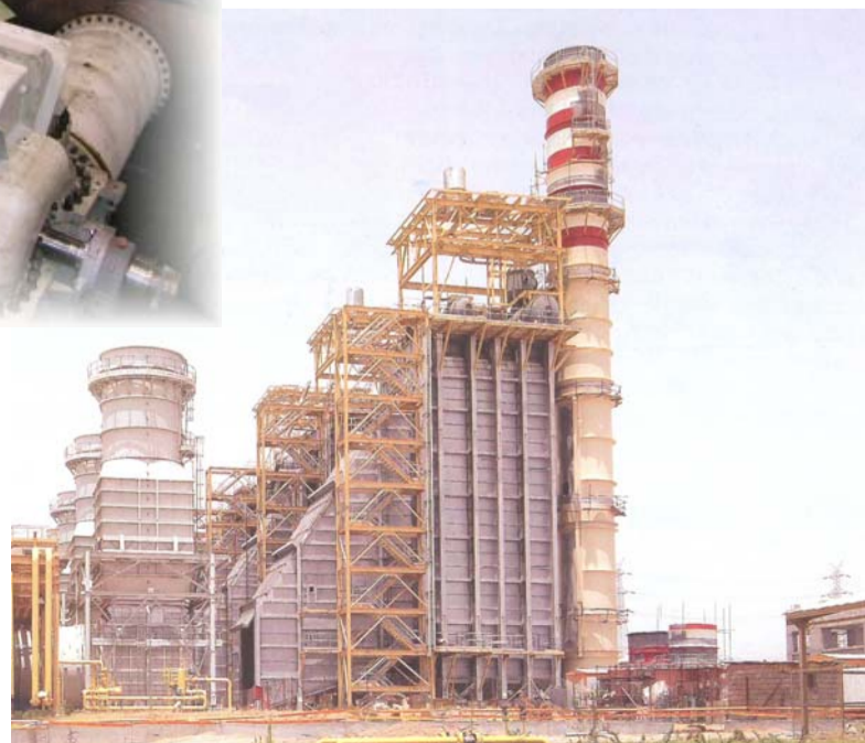
Combined Cycle Plant DAMAVAND - IRAN
